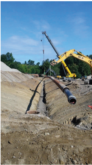
400 feet of encased sewer to reside underneath new SeaTac roadway.
