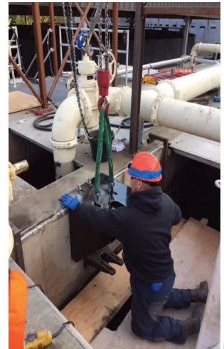
Richie Chapple installing a new bracket he made.
