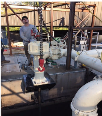
Bryan Asplund operates the slide gate actuator
