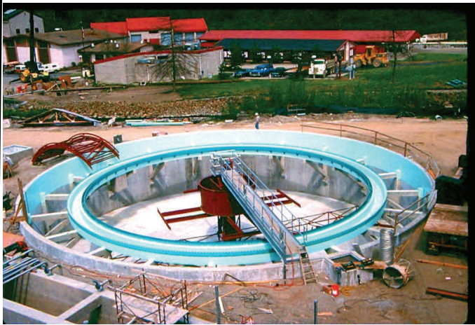
Construction of a secondary clarifier at the treatment plant during Contract 86-2.
